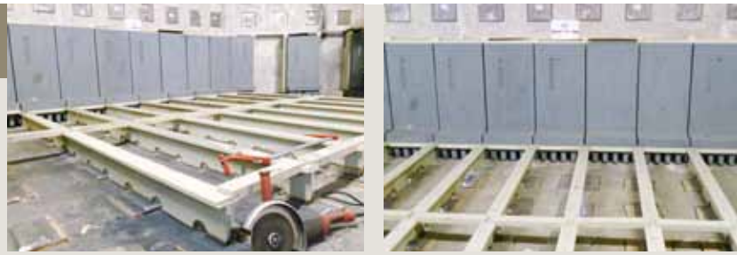
Floor steel structure of the core catcher cooling structure
