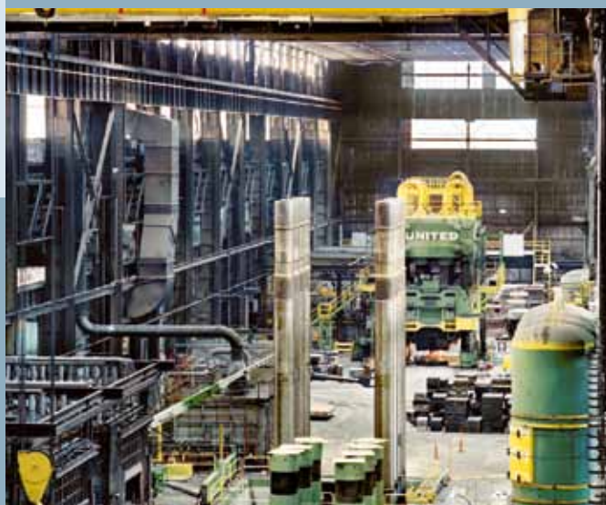
50 K with erected column stands
