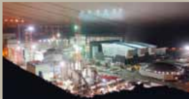
Building site of the new reactor FA3 in Flamanville, France/Atlantic coast
