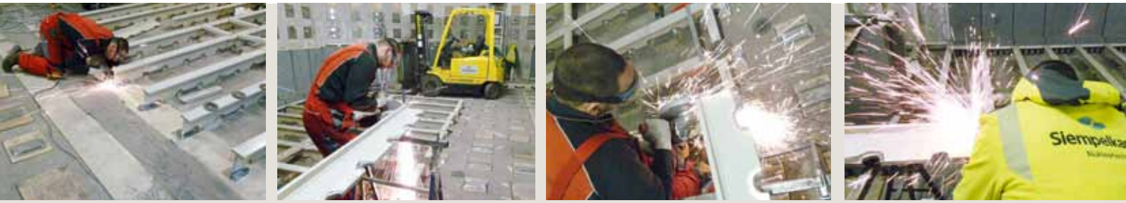
Welding of the single elements for the floor steel structure
