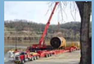
Loading of dryer segments
