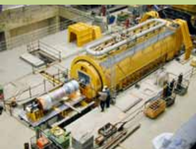
Turbine in a power plant
