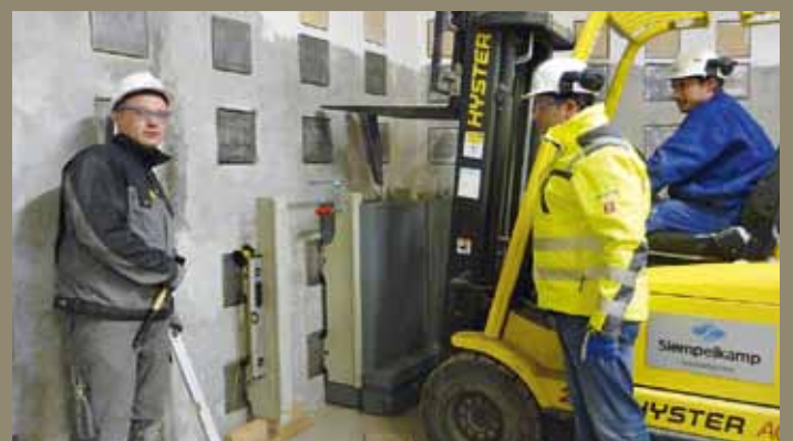
Setting in wall elements in the steel structure
