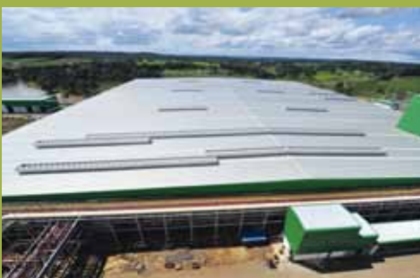
The new factory building – gigantic!
