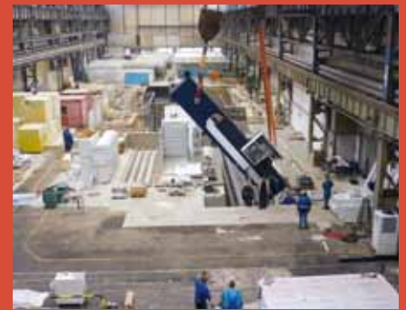
Assembly of the first traveling column drill
