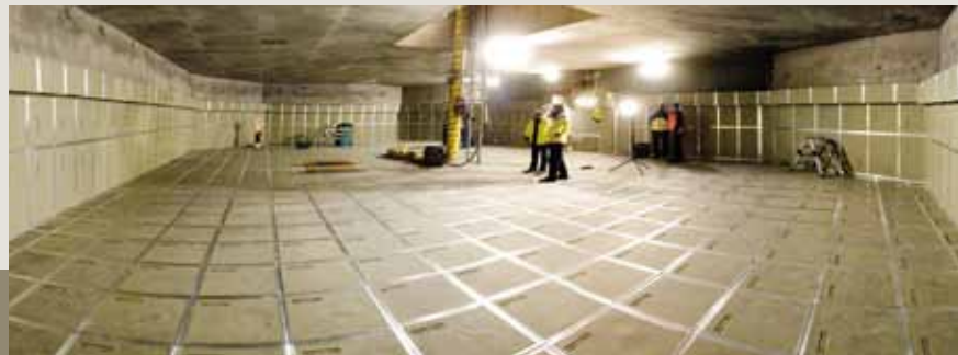
2009: ready-assembled cooling structure of the world's first core catcher in Olkiluoto, Finland
