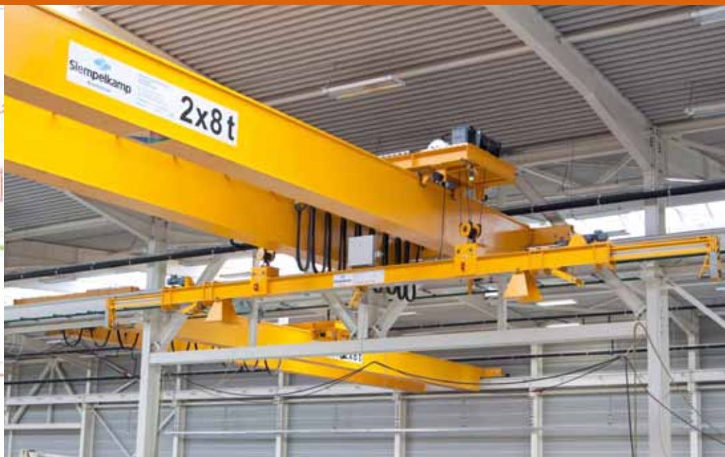
2011: Assembly of a double-girder bridge crane at BUTTING
