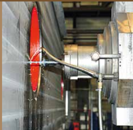
Finishing of the bore holes
