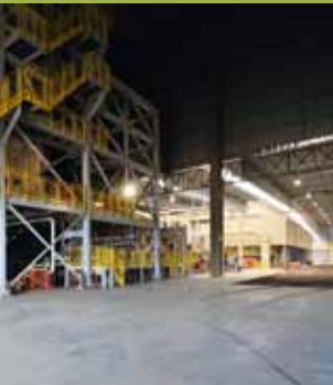
Forming and press line, ContiRoll® with vapor exhaust
