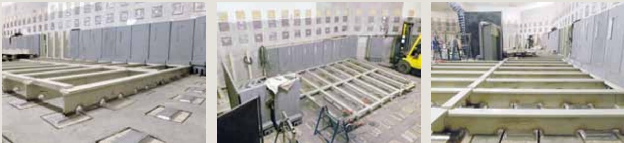
Floor steel structure of the core catcher cooling structure
