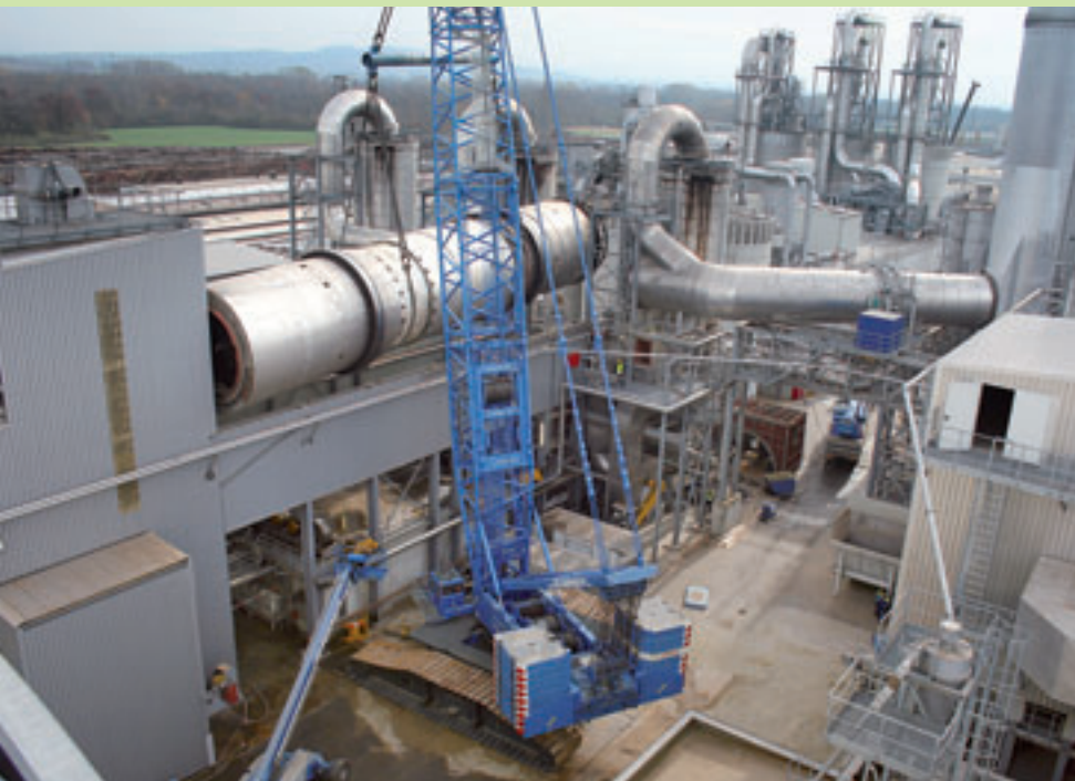
Removal of the old dryer
