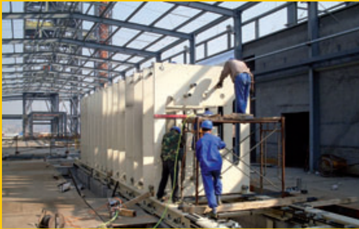
Installation of the frames
