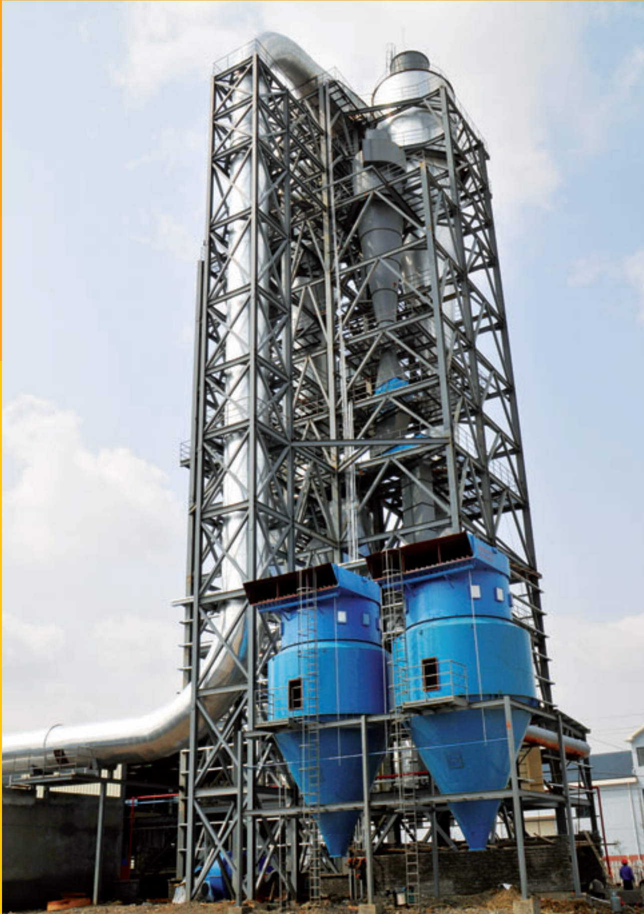
Dryer and cyclone
