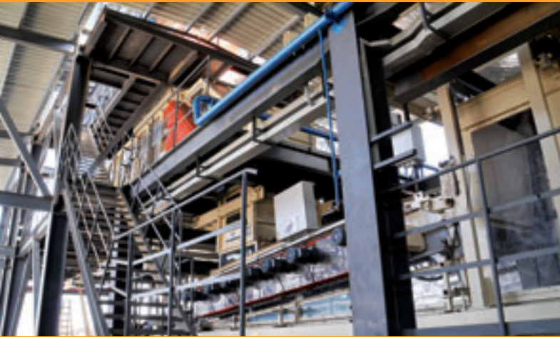
Discharge bunker and former head
