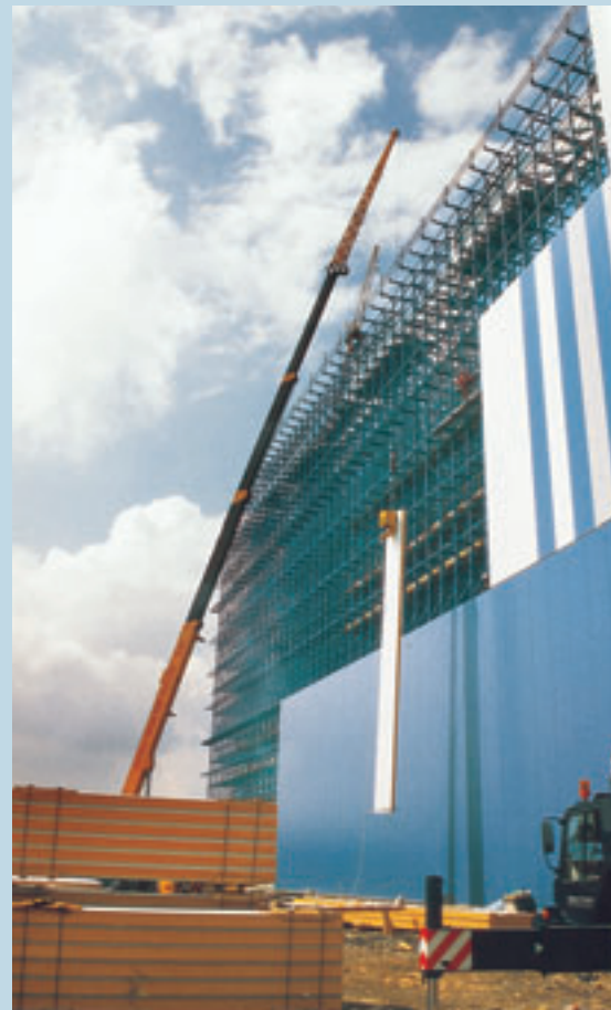
Using the sandwich panels on site
