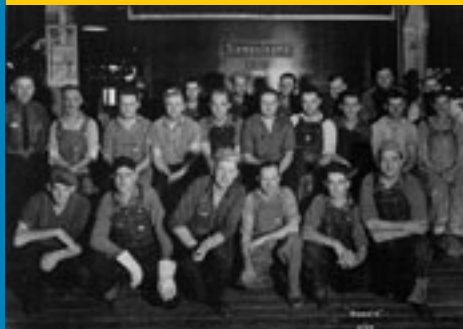
Roddi's Plant, plywood press from 1939
