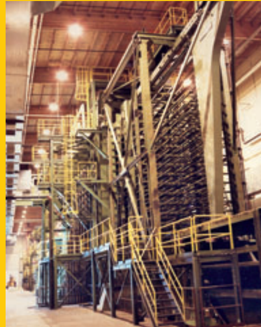
OSB line for Weyerhaeuser, 1982
