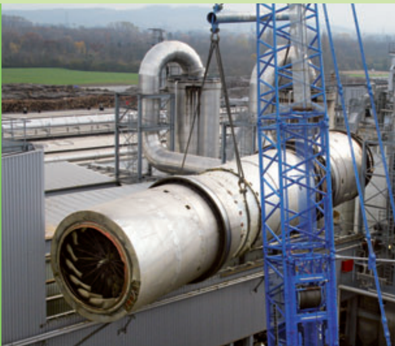
Removal of the old dryer
